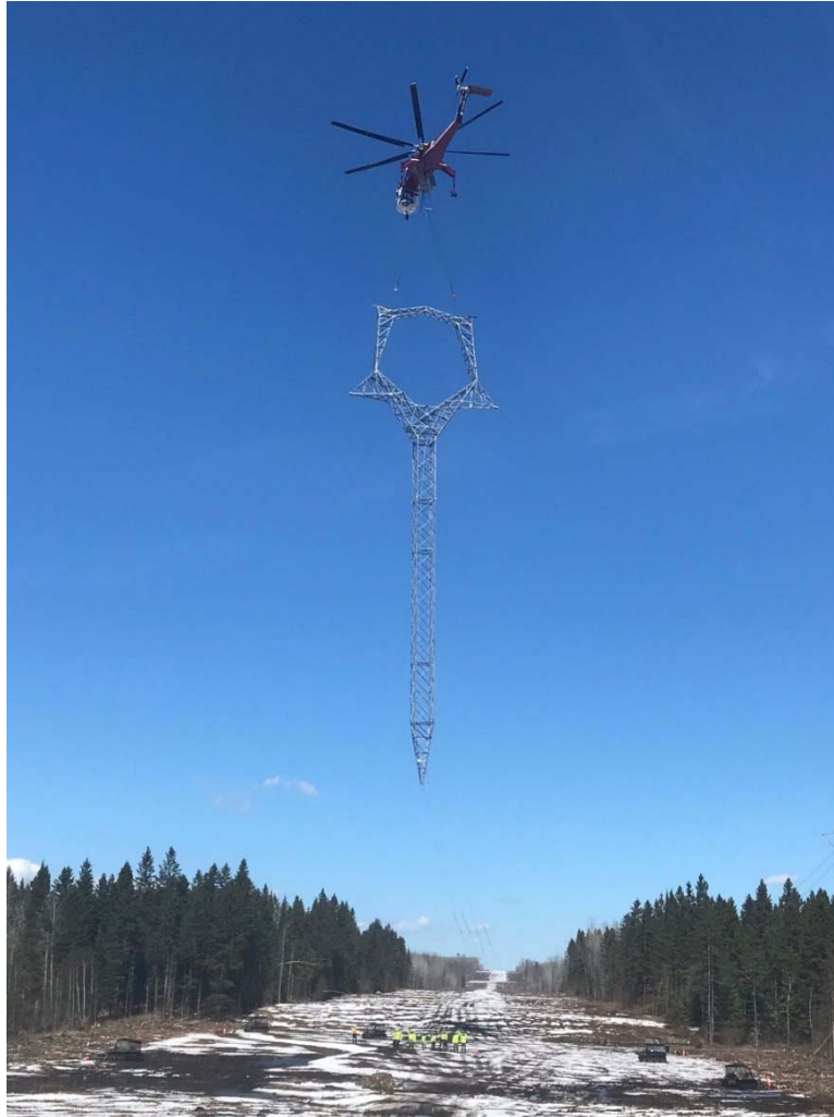
Photo 3: Segment 4 – Tower Setting
